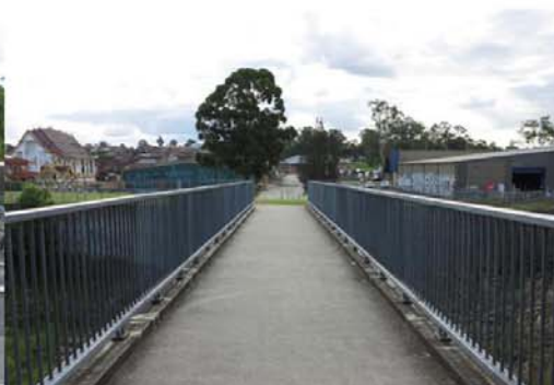
Image 36 – Bridge that connects eastern and western parts of Bonnyrigg Town
