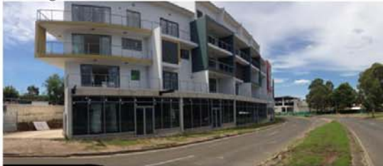
New 6 storey Mixed Use development under construction
