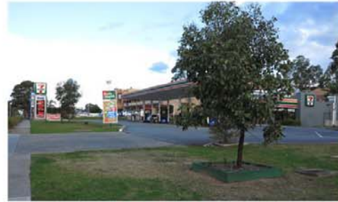
Service Station on Edensor Rd
