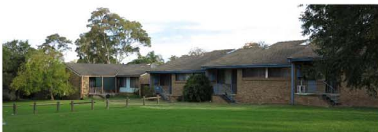
Image 20 Example of original public housing in Bonnyrigg designed using Radburn Principles
